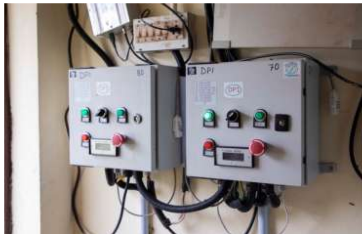
Wireless automatic water flow controllers
