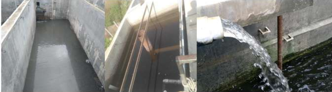
JMR Collection Tank, Settling Tank (after filtration)
